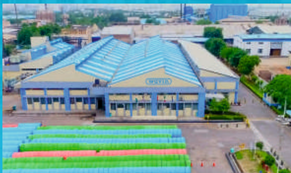
Wavin India, Neemrana Factory
